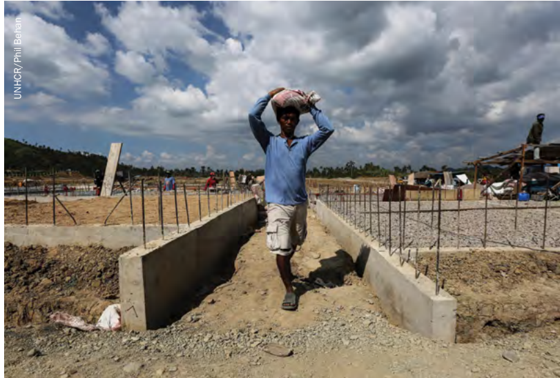
Joel Lacaba working on the construction site for his future permanent home in Tacloban, part of a recovery programme after Typhoon Haiyan, the Philippines.
